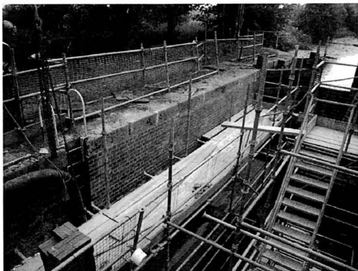
The new brickwork of the chamber wall
