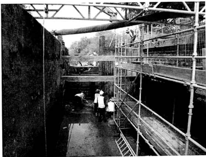
Brickwork repairs to the bottom gate recess
