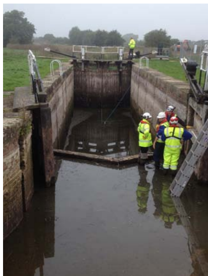
Measuring the top gates
