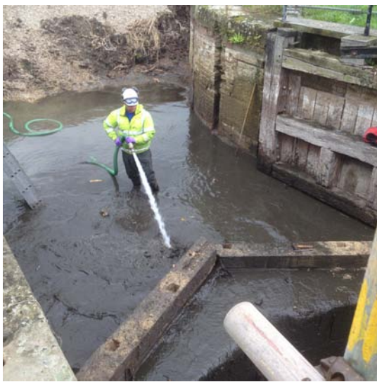
Cleaning above the top gate cill
