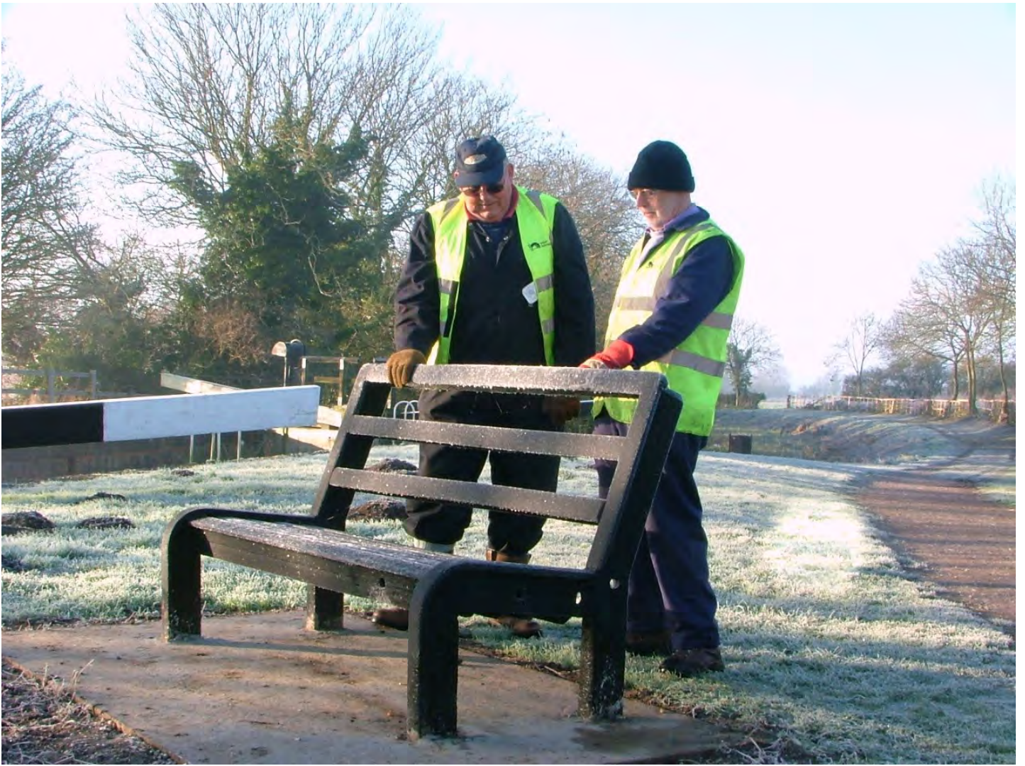
The newly installed seat at Canal Head
