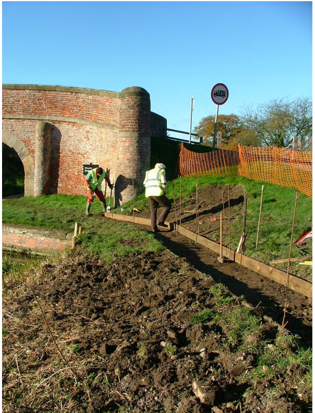
Working on the towpath at Church Bridge photo Andrew Dobson
