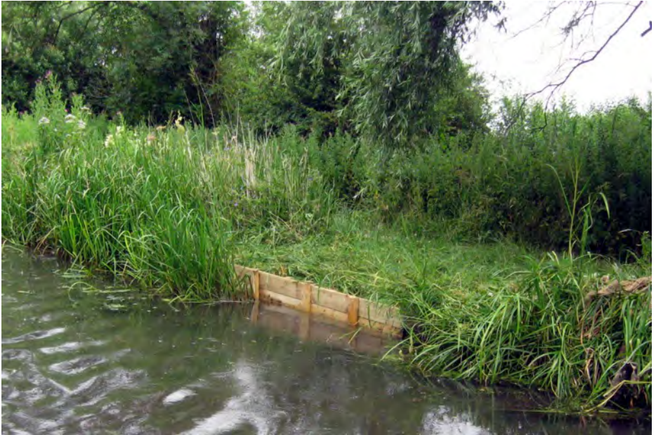
Above: Towpath repairs keep the PCAS volunteers busy throughout the year.
