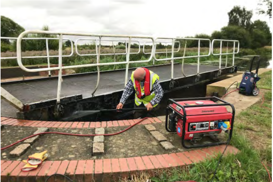
Above: Pressure washing bridge No6 prior to repainting.
