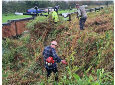
Above: Brambles and overgrowth being cleared, before the dredging.
