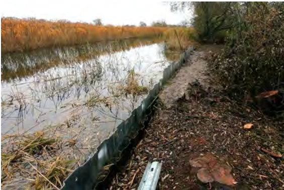
Left: With the reeds cut back and the new piles in place, notice how wide the canal is at this point..
