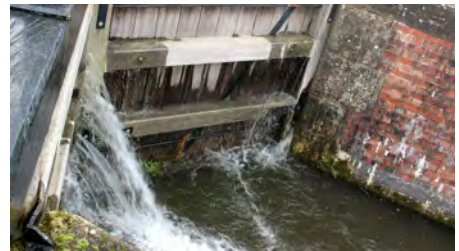
Left & Right: The leaking bottom gates at Coates Lock, which will be dealt with in the next stage of restoration.
