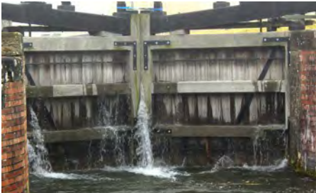
Left & Right: The leaking bottom gates at Coates Lock, which will be dealt with in the next stage of restoration.
