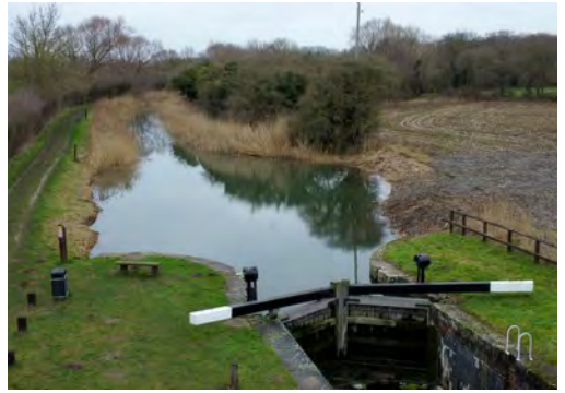
Above: The now visible winding hole at Coates Lock photographed on the 11th January 2024.
