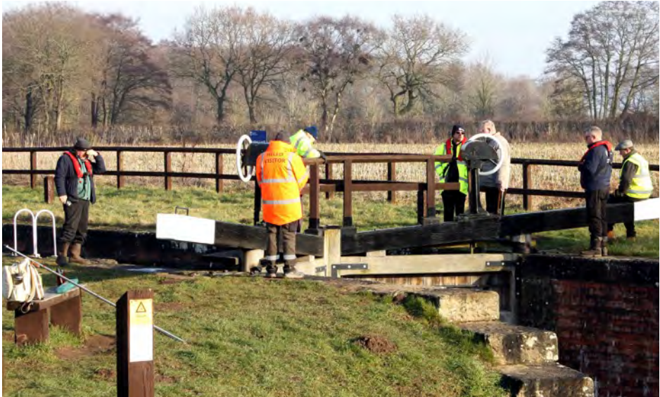
Above: PCAS committee members, along with CRT engineers, inspect Coates Lock as part of the project to re-open the Bielby to Coates section.
