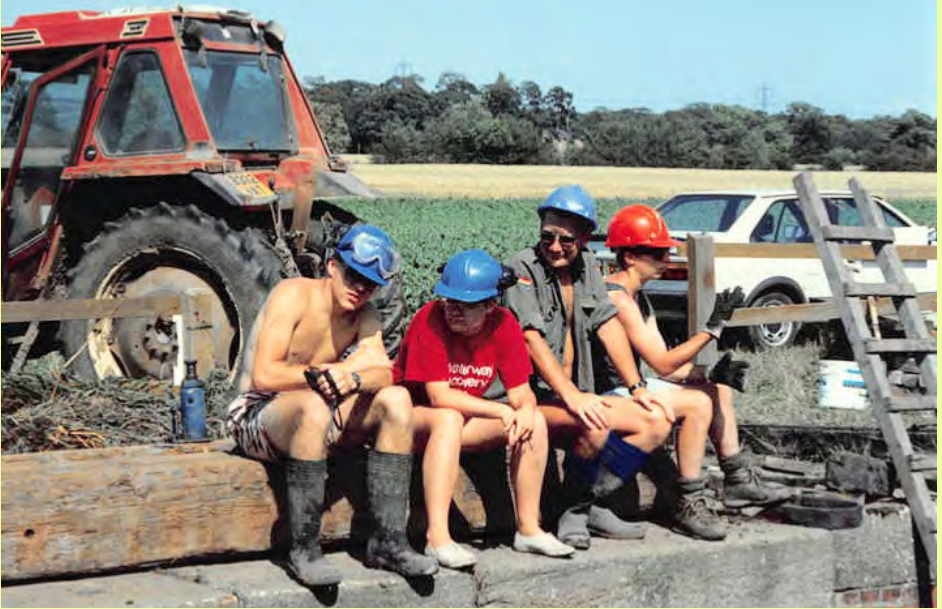
Above: Members of the Waterways Recovery Group take a break at the Walbut lock restoration on the 19th July 1992.
