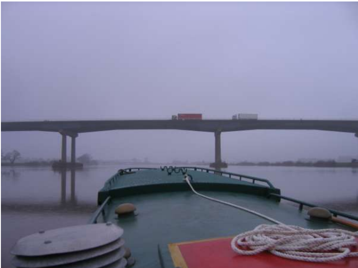
Approaching the M62 viaduct
