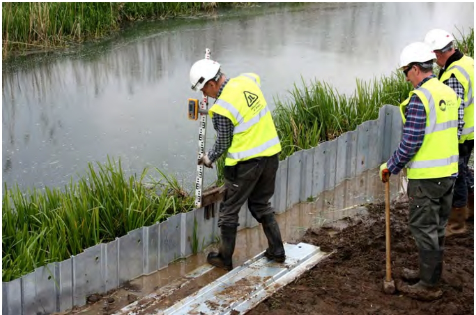
This page: Work has now commenced on installing the top and bottom landing stages at Thornton Lock. PCAS working party members are seen installing the bottom landing stage on the 30th April. Work was well advanced when the lower image was taken on the 1st May. Photographs by Malcolm Slater
