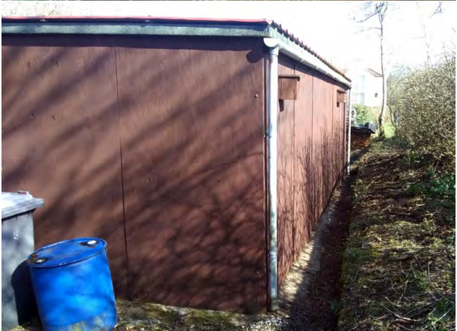
This storage shed at Canal Head was erected by volunteers in May & June 1982 ( top picture ) and has lasted 40 years! The shed received a fresh coat of timber treatment on the 8th March this year. The drainage channel at the rear of the store was also cleaned and cleared of debris. Note the two bird boxes affixed to the rear wall.
