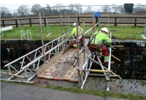
Specialist scaffolding contractors installed a bridge and steps down into the lock.
