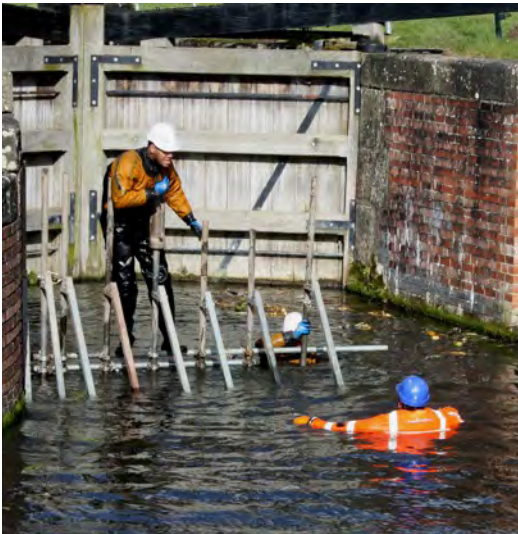
Above & Left: The steel framework being installed.
