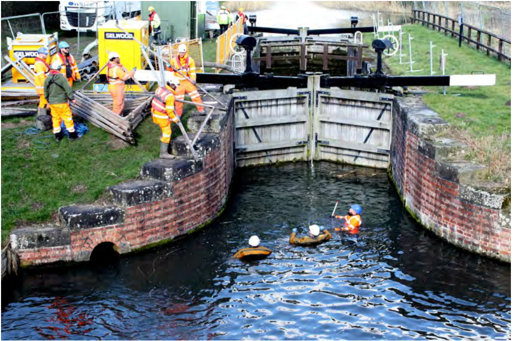
Above: Workmen preparing to install the lower fabric dam.
