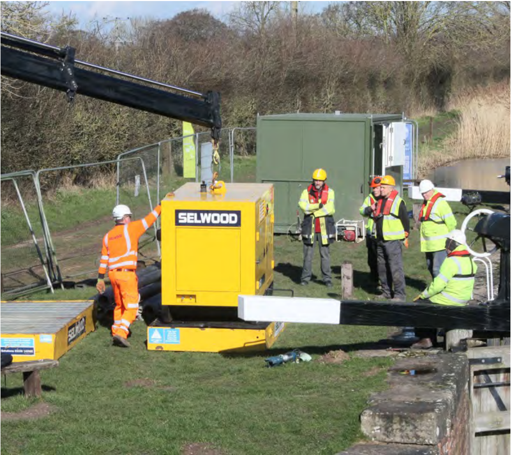
Above: Pumps were hired to keep the lock drained - the main pump was lowered into position.
