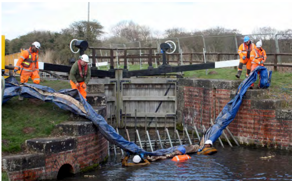
Above & Below: The fabric is rolled across the metal frame to create the dam.
