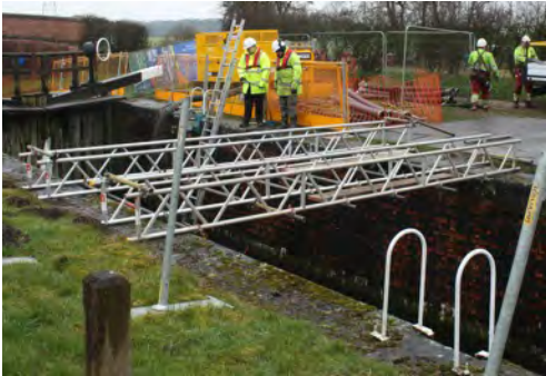
Specialist scaffolding contractors installed a bridge and steps down into the lock.
