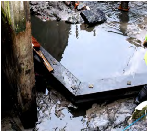
Left: The problematic lower cill was finally exposed. Plans to seal below them were to be undertaken the following day.
