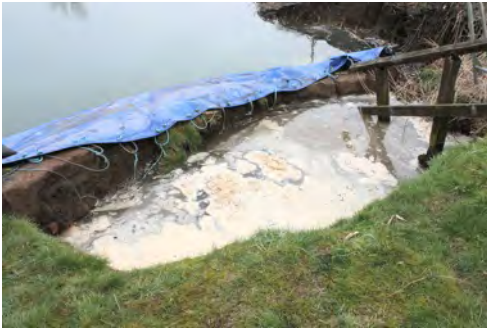
Above & Left: The lock chamber now filled with water and the collapsed wing wall.
