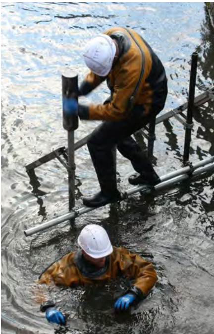
Above: Workmen preparing to install the lower fabric dam.
