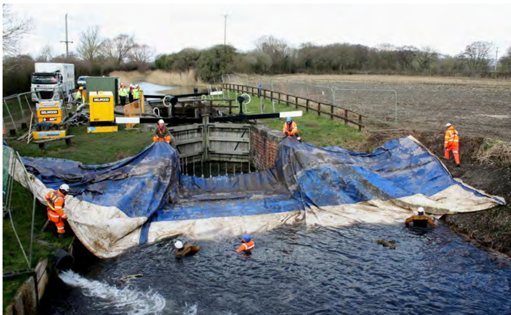
Above & Below: The fabric is rolled across the metal frame to create the dam.
